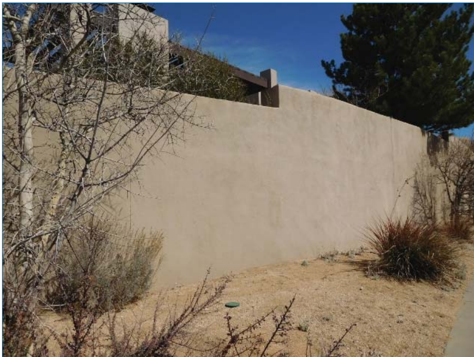
Typical common area stucco wall
