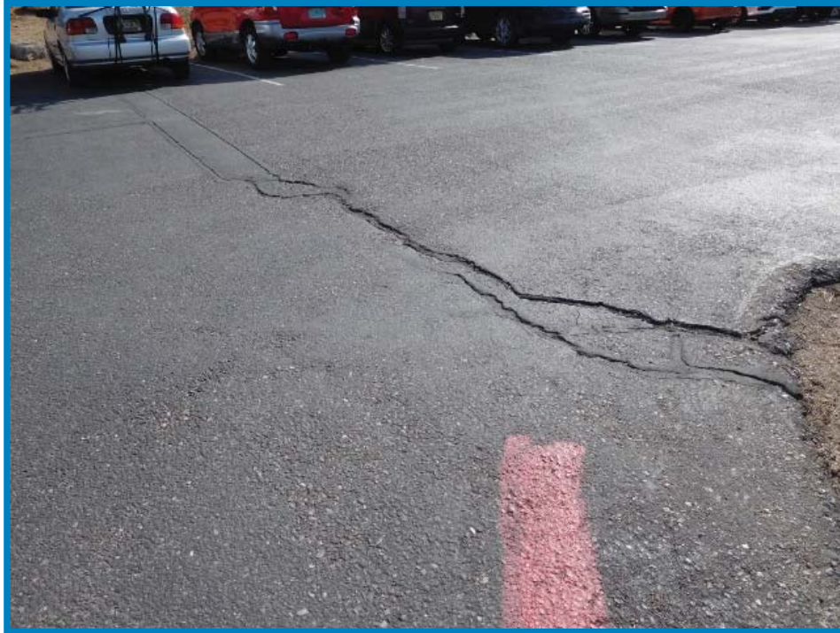
Typical parking lot asphalt at Michial Emery trailhead
