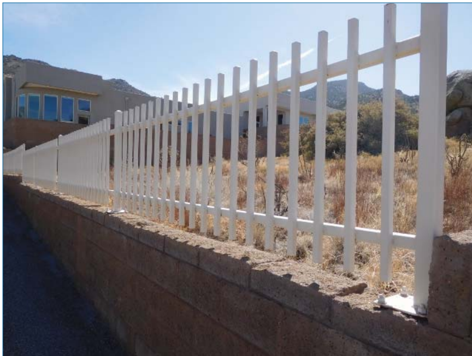
Typical metal perimeter fencing
