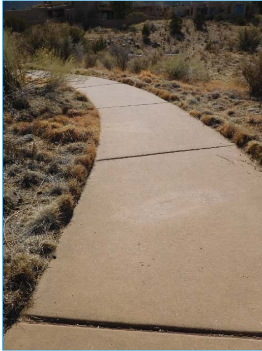
Typical concrete walkway
