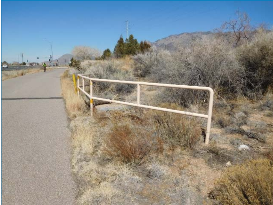
Typical metal piperail fencing
